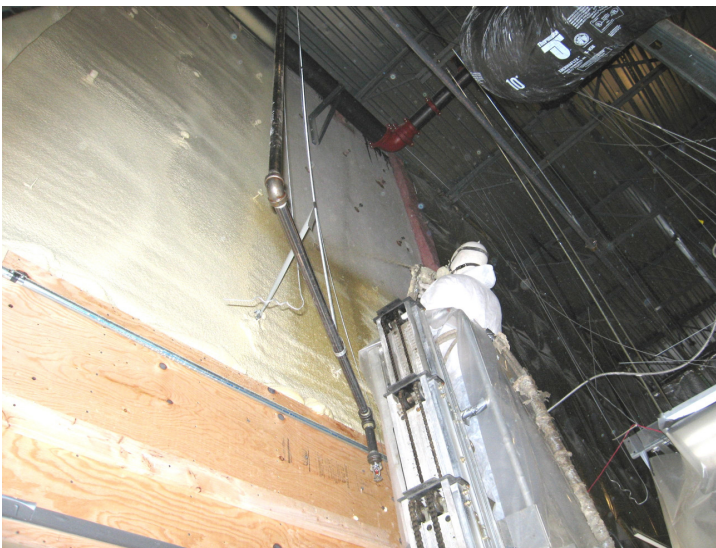
SR spray foam being applied to inside
