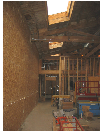
2. Installation of sheathing and SR Foam™
