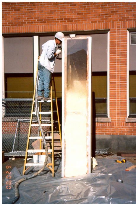
3. SR Foam™ filling wall cavity
