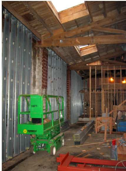
1. Installation of metal studs
